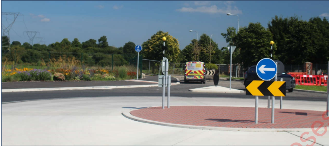
Plate 11-28 A roundabout on Moyglare Hall Road, where the proposed MOOR and Moyglare Bridge will link the Existing Road Network in County Kildare
