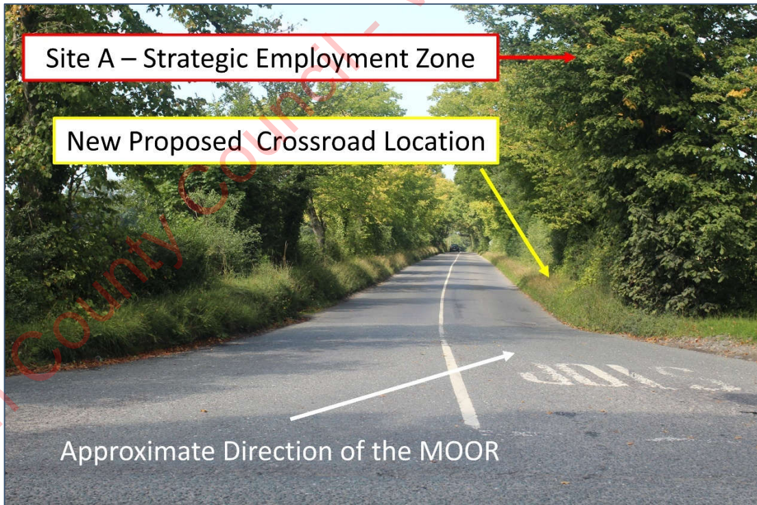
Plate 11-14 View west-north-west along the L2214-3 Local Road from the existing junction with the R157.
